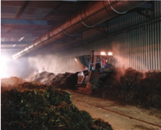
Composting of residual waste at New Earth Solutions' MBT facility in Dorset, which diverts over 80 per cent of biodegradable municipal waste from landfill
