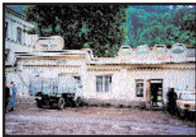
Borjomi mineral water bottling factory
