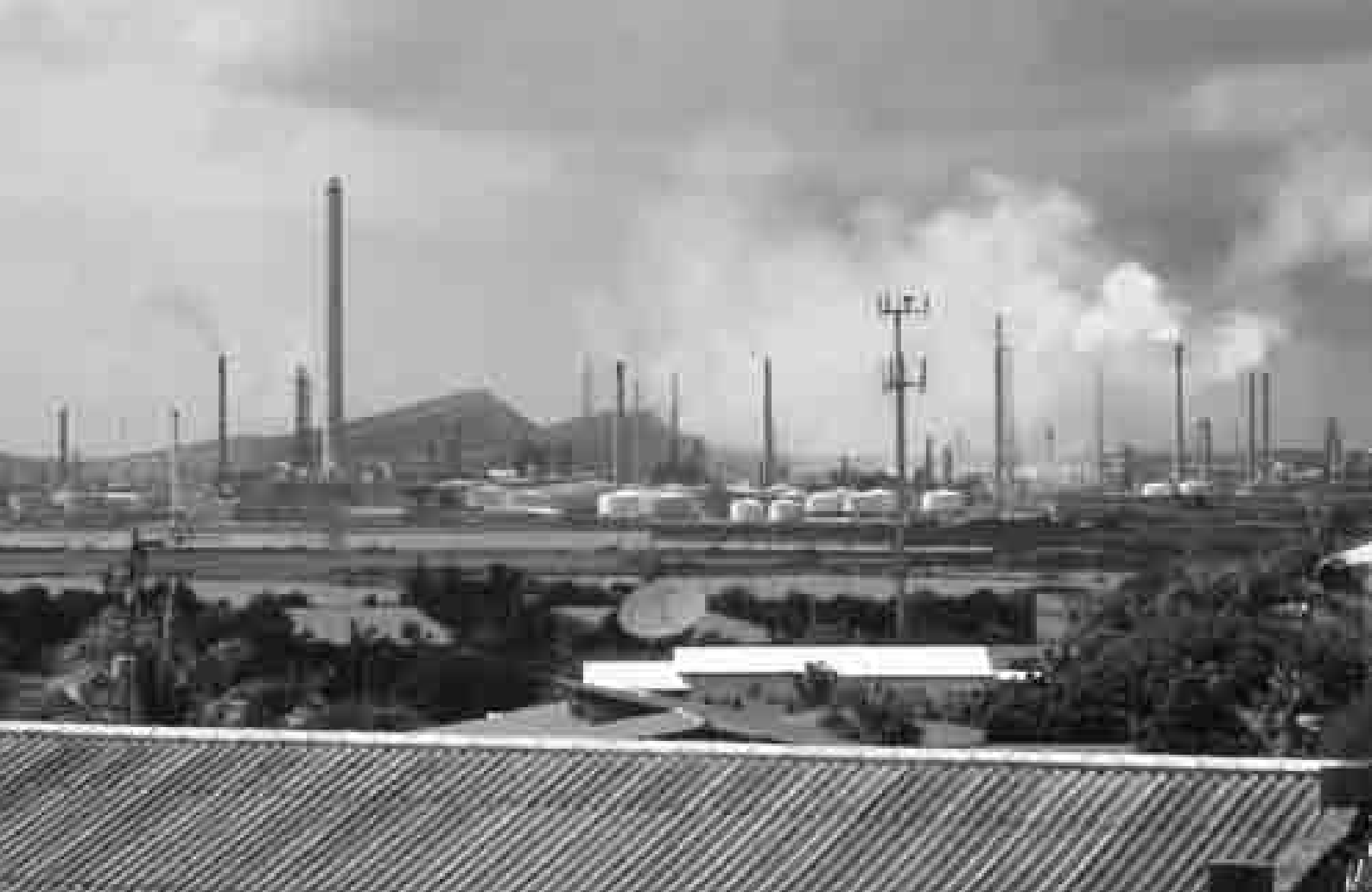
The former Shell refinery located dangerously close to the residents of Curaçao. (Denny Larson/GCM)
